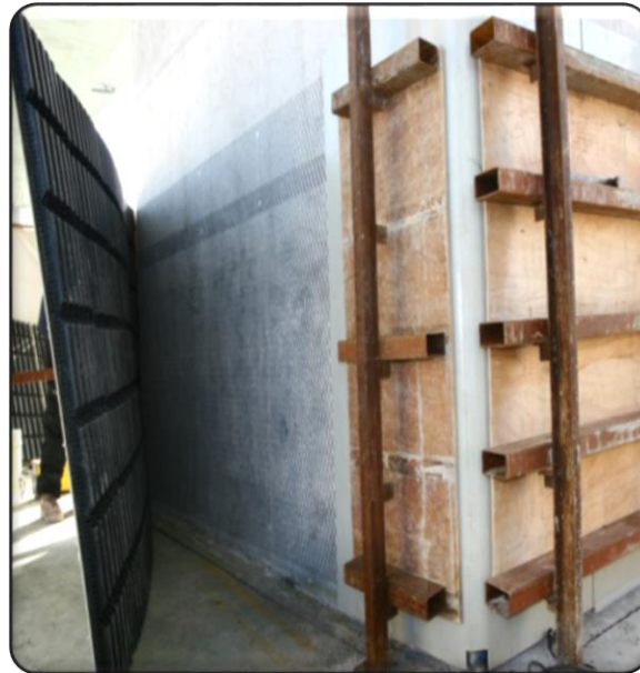
Installation of FRP Cover
