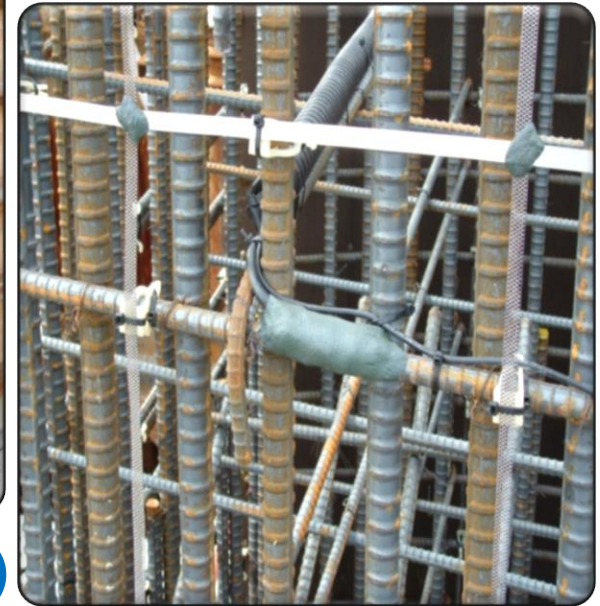
Mold for Work Process
