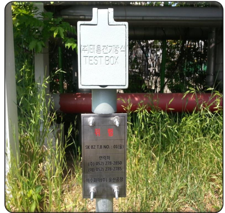
Test box Installation
