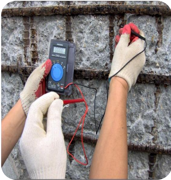
Corrosion Investigation and Inspection
