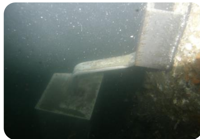
Installation of Al-Anode
