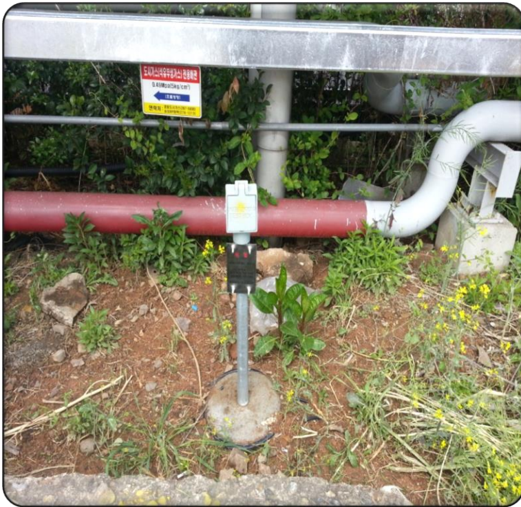
Test box Installation
