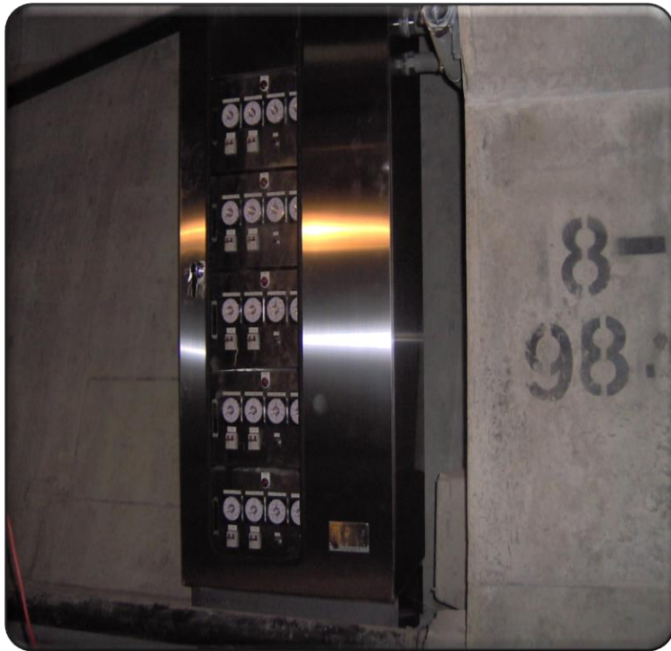
Installation of Rectifier
